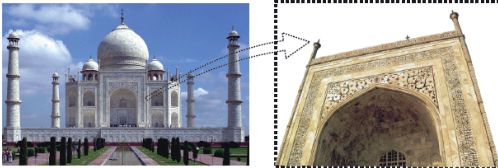
Figure 16.17: Taj Mahal and its corroded door
